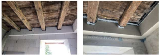
Fig. 6: Upper floor: wooden beams
