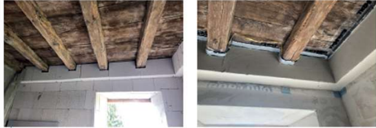
Fig. 6: Upper floor: wooden beams
