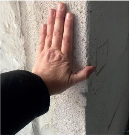
Fig. 3: Mutipor panels thickness of 140 mm
